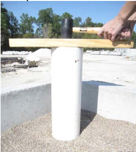
Figure 3: Hammer pipe into media
